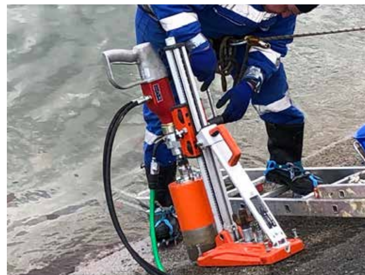
MAR IN CO d.o.o. PODVODNA DELA
